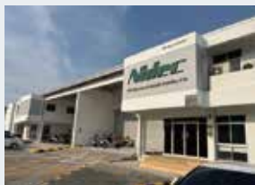
NIDEC ADVANCE TECHNOLOGY (THAILAND) CO., LTD.
